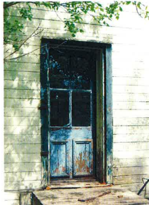
Figure #5: Original rear door
