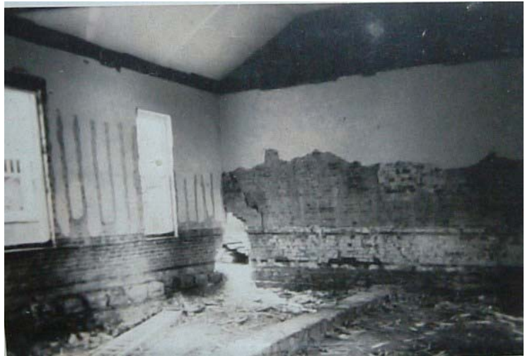
Damaged back wall of Town Hall, July 1975
