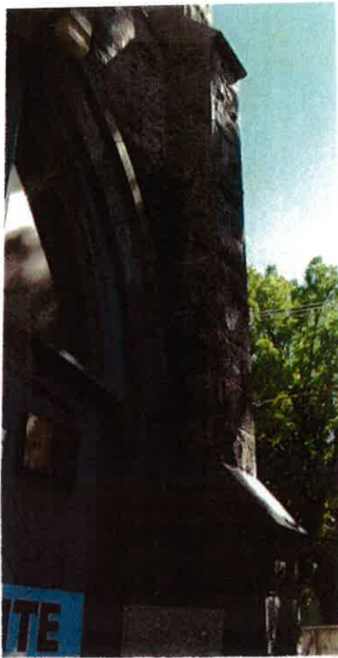
Typical Wall Buttress (not a flying buttress)
