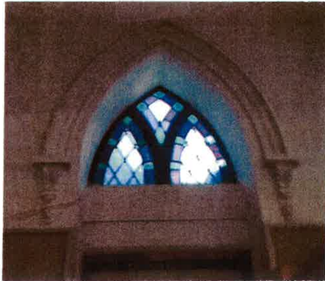
Arched pointed window
