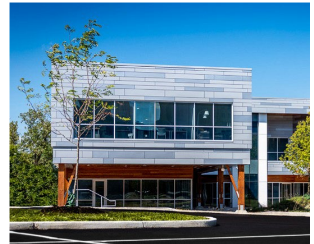
High quality architectural finishes should be visible from the 400-series highways (Photo: Hixson Inc.).
