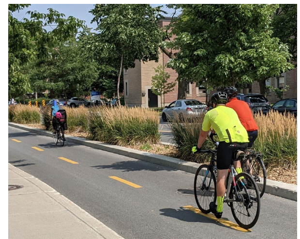
Bicycle lane with planted median.
