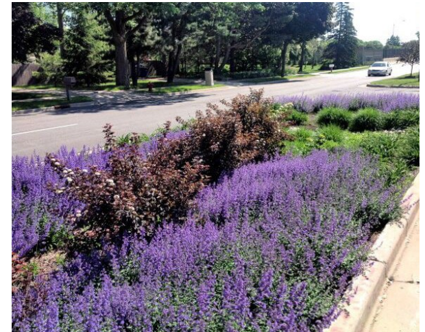
Bioswale in green boulevard (Photo: MMSD).
