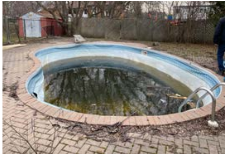
Stagnant water in an inground pool
