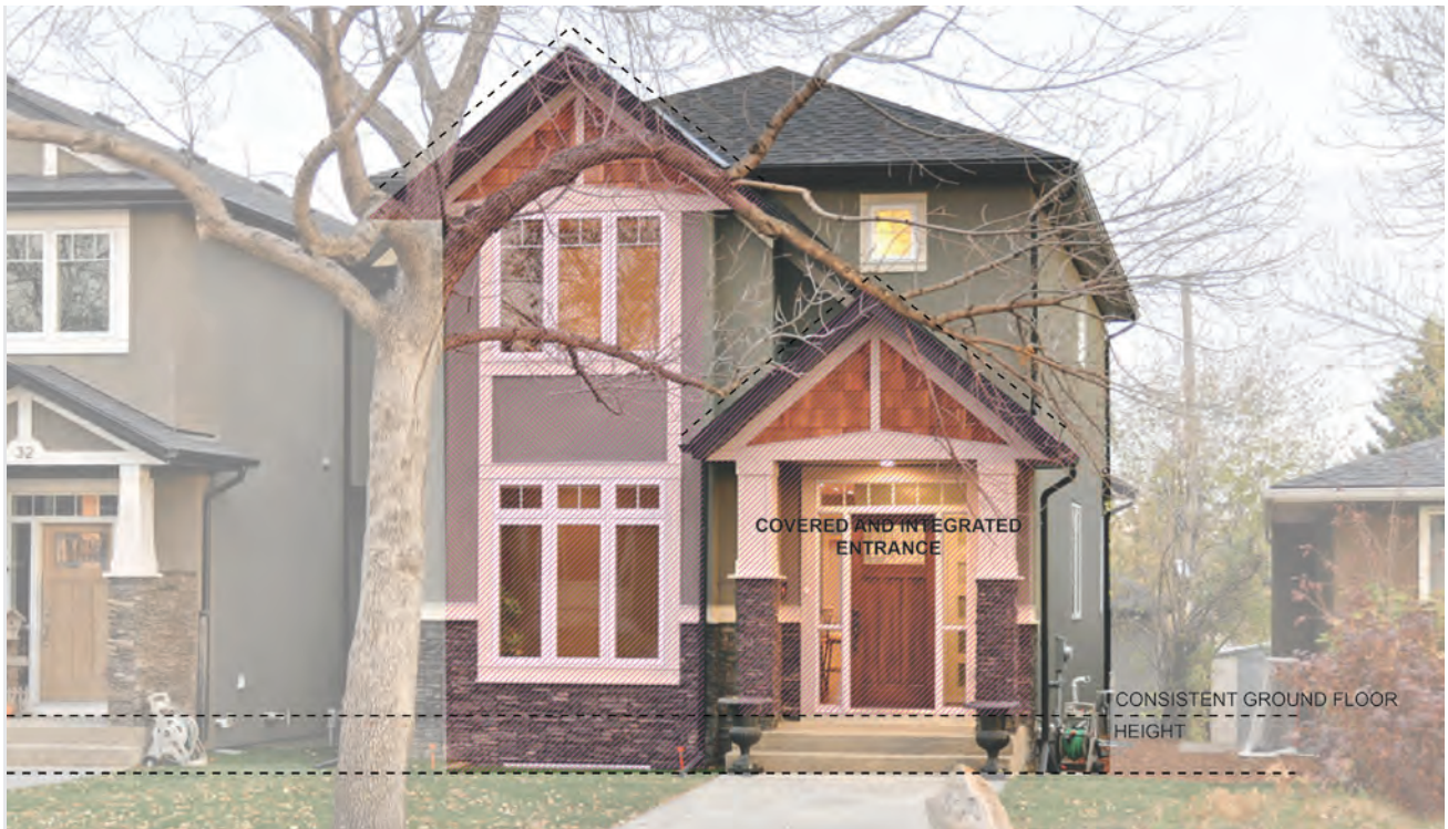
Figure 29: Integration of a covered entrance within the overall building design
