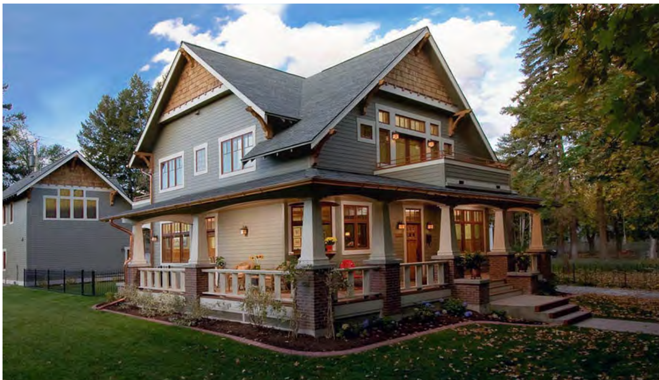
Figure 35: Mix of building materials including cedar accent shingles, wood siding, and brick masonry columns
