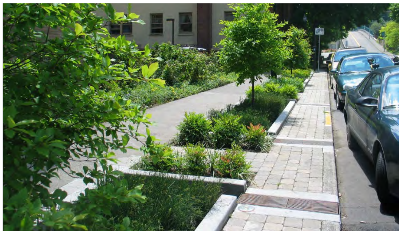
Figure 54: Planted bioswale to mitigate stormwater runoff
