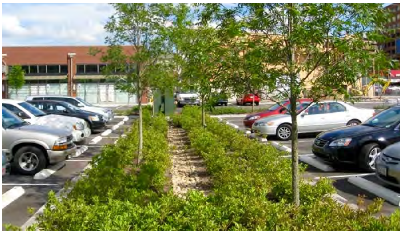
Figure 53: Planted bioswale in between parking lanes to mitigate stormwater runoff with surface parking lots
