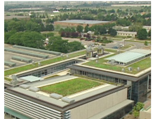
Green roofs can provide habitat for some animals, reduce stormwater run off, and reduce the urban heat island effect.
