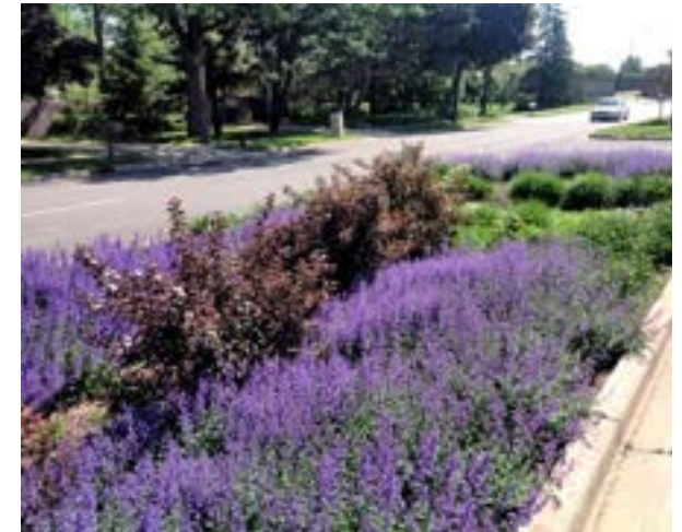
Bioswale in green boulevard (Photo: MMSD).
