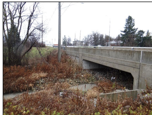
Plate 4: Mullet Creek passing under Winston Churchill Boulevard, looking southwest (ASI 2020)
