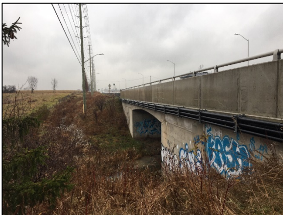
Plate 9: Bridge along Steeles Avenue, looking east (ASI 2020)
