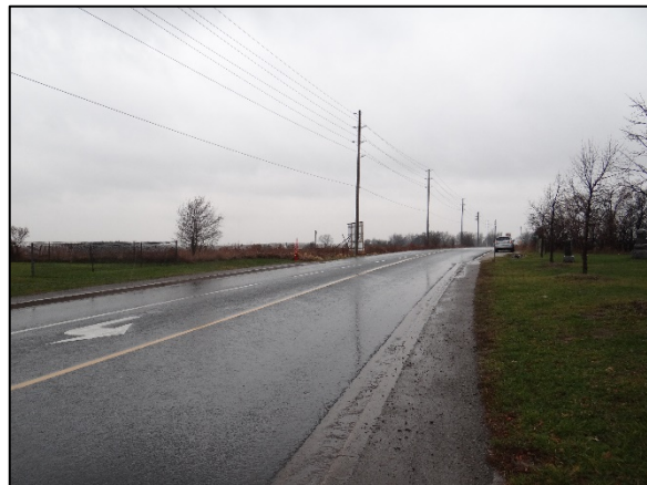
Plate 16: Looking north along Eighth Line (ASI 2020)
