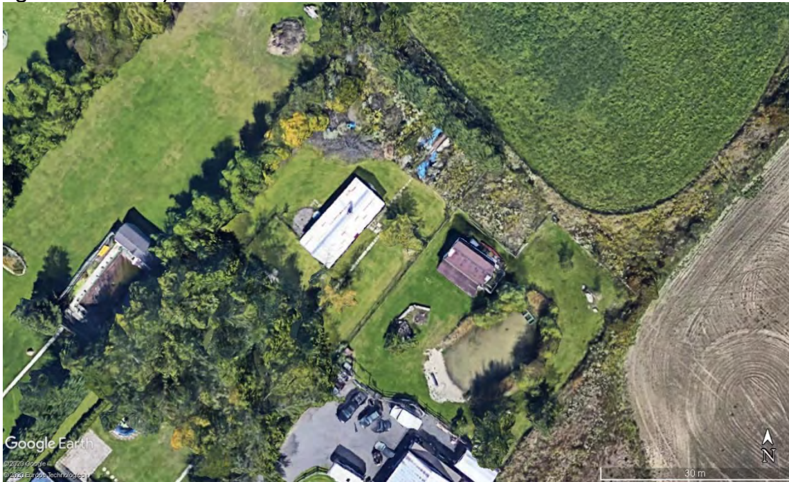
Agricultural Facility #20 and #21
