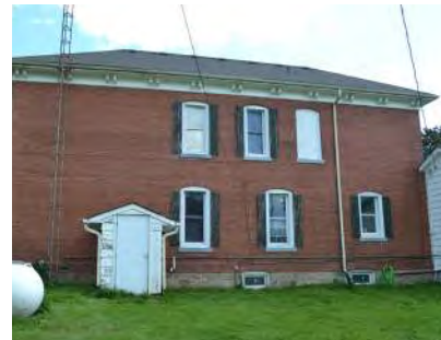
Figure 5 - Reinstatement of Wooden Cellar Entrance
