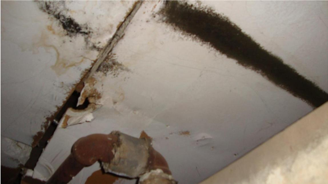
**Photo 13: View of mould on ceiling -79 Main Street S building**
