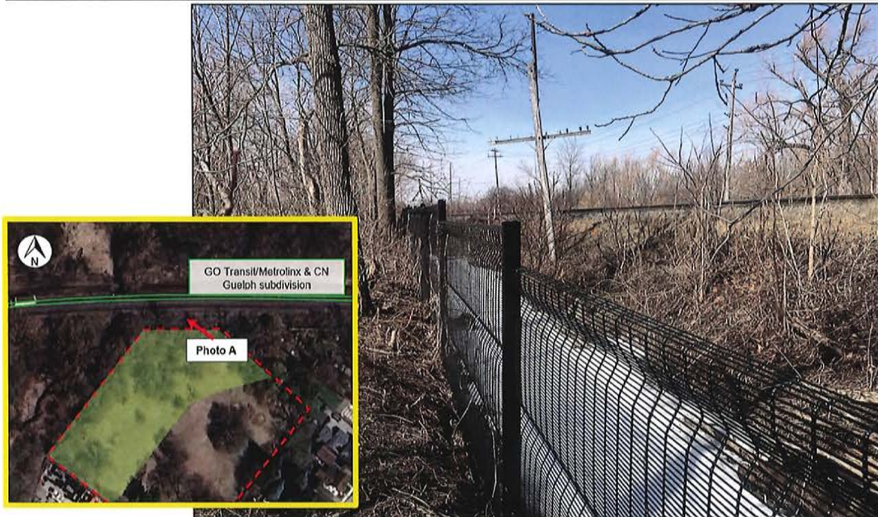
Figure 2: Photo A taken at the mutual property line showing the existing elevation of the track (right) in relation to the Site (left). Existing high-security fencing is also present at the mutual property line. Source: Field Photos taken 25-Mar-2026.
