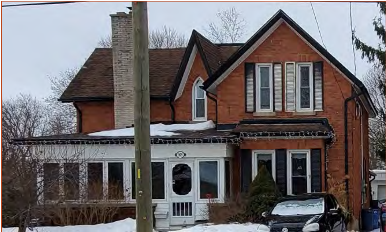
Photo 11. View northwest of 105 Bower Street.
