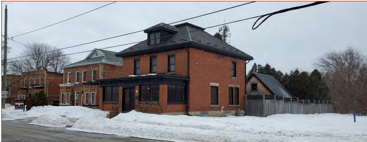
Photo 8. View northwest of the south and east elevations of 93 Bower Street.
