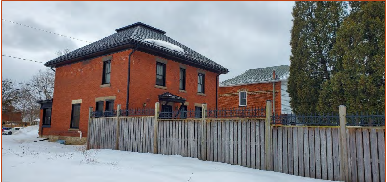
Photo 10. View south of the east and north elevations of 93 Bower Street.
