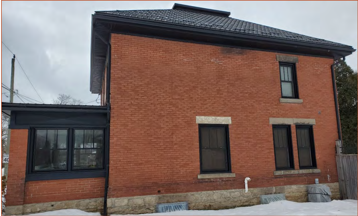
Photo 9. View southwest of the east elevation of 93 Bower Street.
