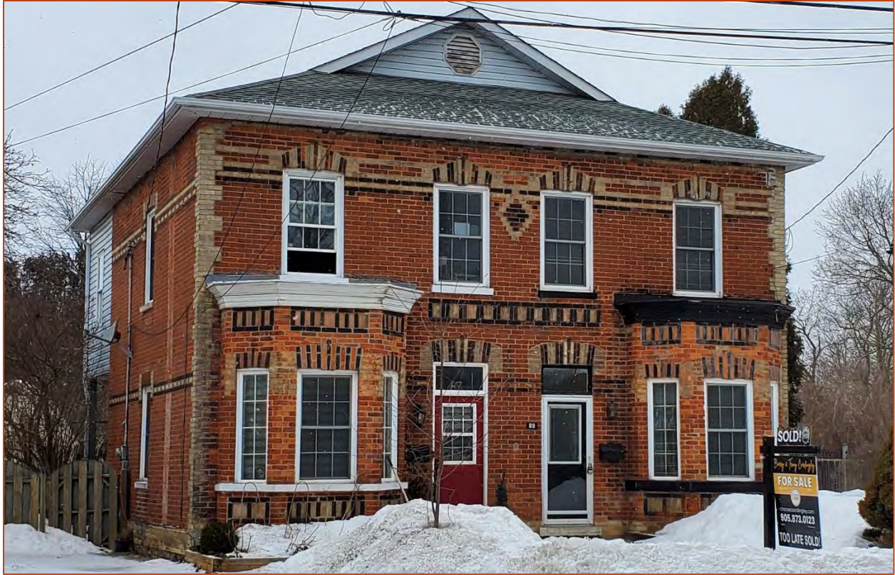
Photo 6. View northeast of 87 and 89 Bower Street.
