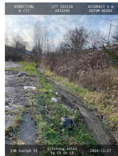
Photo 2: Location of ditching, looking west
