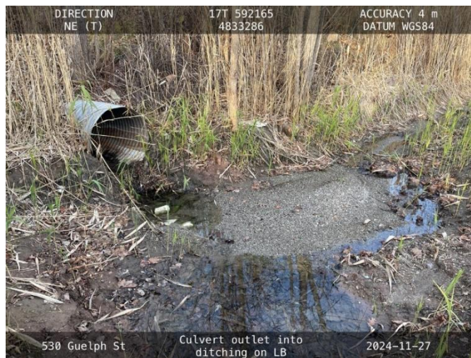
Photo 1: Culvert under Guelph Street to Credit River on Client Property
